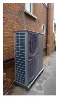
In practice the SCOP will vary a lot according to the outside air temperature and the water temperature going into the radiators. With outside air at 10degC and radiators at 40degC, our heat pump will achieve a SCOP of up to 4.5. But with outside air at minus 15degC (rare in Orpington!) and radiators at 55degC (maximum output temperature) the SCOP would drop to around 2.0.
