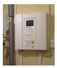
The other reason you need to increase insulation is down to the way a heat pump is programmed. A gas CH system has a simple programmer, typically with four ON/OFF periods each day. It tends to be set to turn off at night, and come on just before you come down for breakfast. It *assumes* the house will cool down at night, because of poor insulation, and then need to be heated up quickly with very hot water pumped through the radiators.
